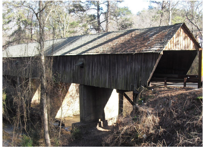
Concord Covered Bridge (Photo c/o ConcordCoveredBridge.org)
